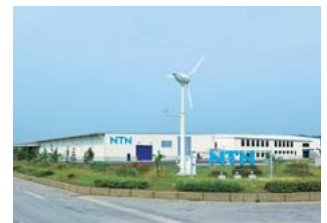
Wind power generator (NTN Houdatsushimizu Corporation)
