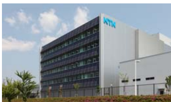
Solar power generator (Elemental Technology R&D Center)
