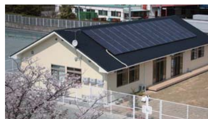
“Bear Kids Land” building with installed solar panels
