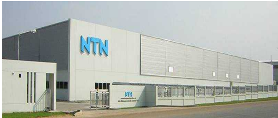
NTN MANUFACTURING (THAILAND) CO., LTD. Exterior view of fluid dynamic bearing production plant
