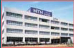
Kuwana Engineering Center (Mie, Japan)
