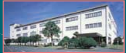
Iwata Engineering Center (Shizuoka, Japan)
